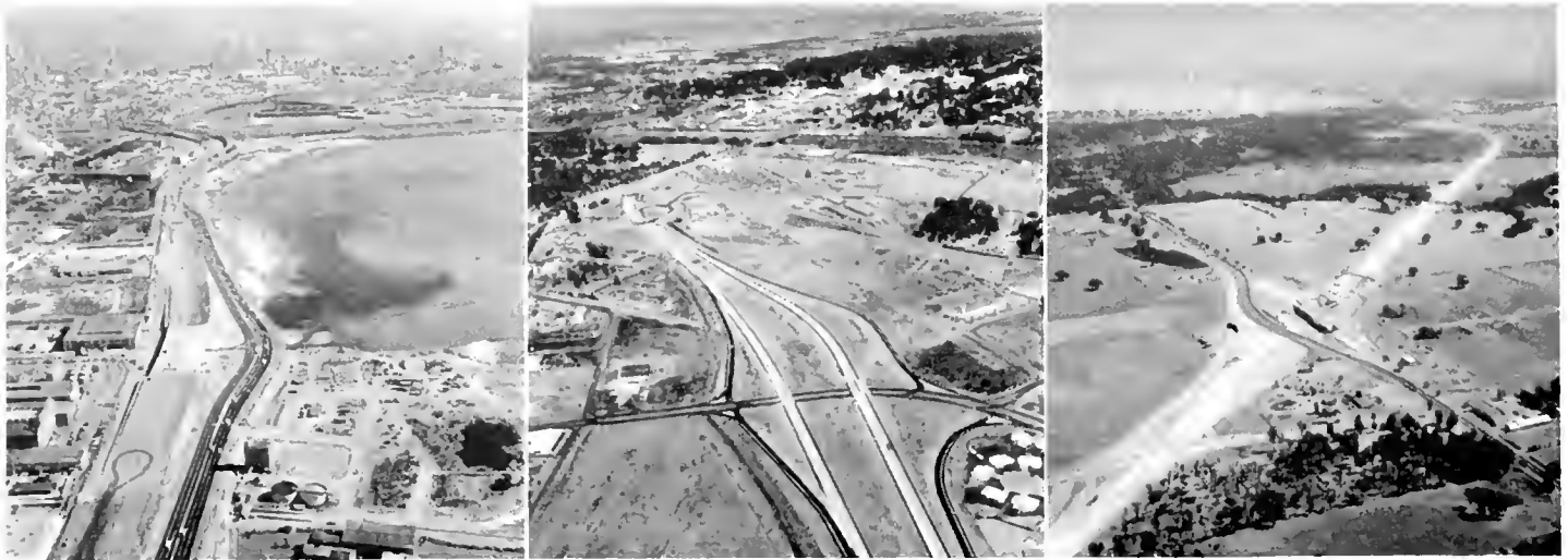
LEFT: Eastshore Freeway, US 40, looking south toward downtown Oakland, showing construction under way on Powell Street separation structure. CENTER: Looking west along the recently opened West Sacramento Freeway. RIGHT: Near Sacramento-Placer county line traffic an existing US 40 crosses construction zone along new freeway route. View is east toward Roseville.
